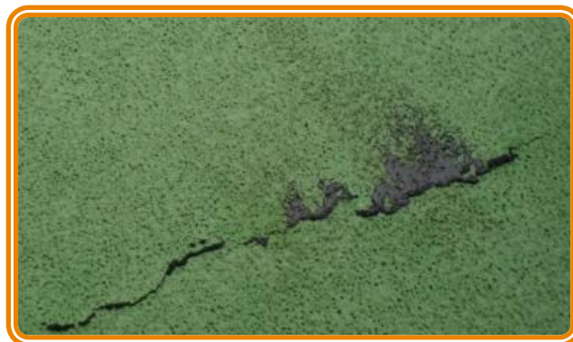
LBE leeching through splits in the acrylic surface
