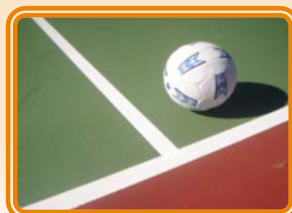
Well installed line marking – crisp & sharp edges
