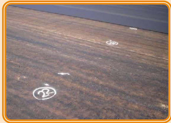
Surveyed and marked
