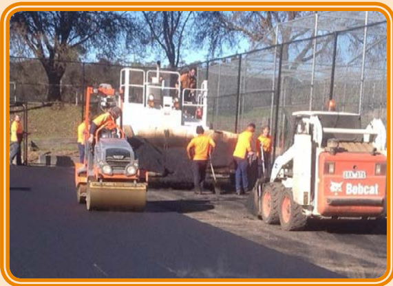
Asphalt paving machine
