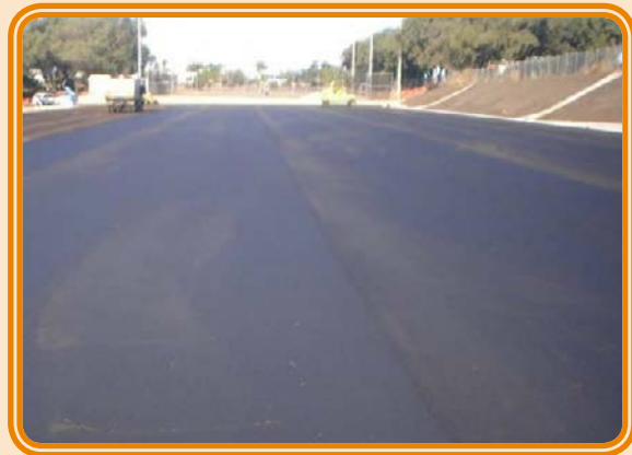
Asphalt laid in runs
